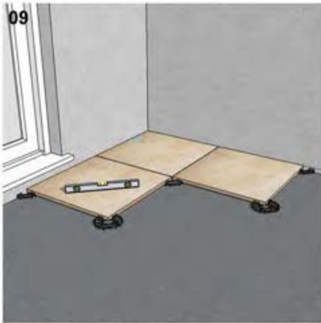
09 - Lay the adjacent paving supports and slabs. Cut the edge paving supports and retain tabs to the edges as outlined in 6 above. Using a spirit level ensure each slab is level as the work progresses. Continue laying the paving by laying adjacent slabs in a diagonal pattern as indicated in 10 - 14.
