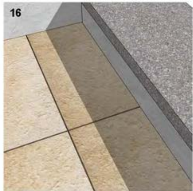
16 - Continue laying the pedestals and cut slabs in the same manner to all remaining edges requiring cut slabs.
